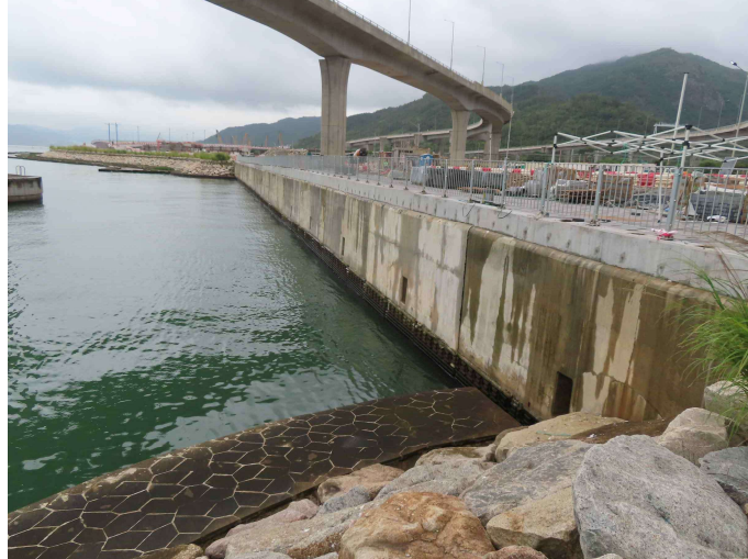
General View of Vertical Eco-shoreline
